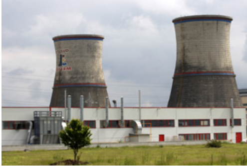
Fig. 1 The cooling tower from the area of CET Timișoara South
