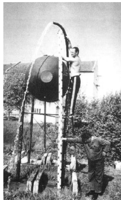
Fig.8 Storage tank at about 4m above irrigation ground level with a leveling staff
