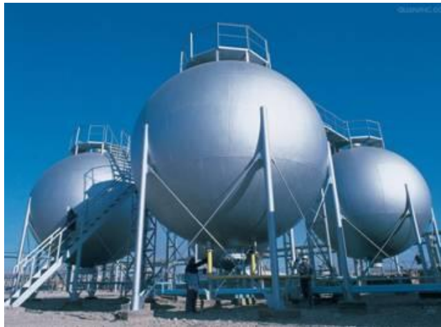
Fig. 2.5. Recipient sub presiune sferic [ http://3d-labs.com/Pressure%20vessel%20e-book-Types.html ]
