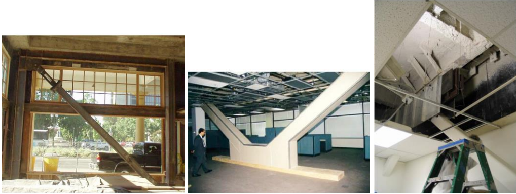
Fig. 2-8. Installed VE solid dampers on Hotel Stockton, LAPD Recruit Training Centre and San Mateo County Hall of Justice [10]
