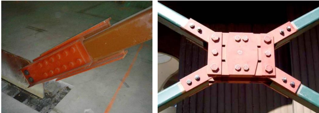
Fig. 2-4. Installed friction dampers on Monterey County Government Centre [11] and on Patient Tower [12]
