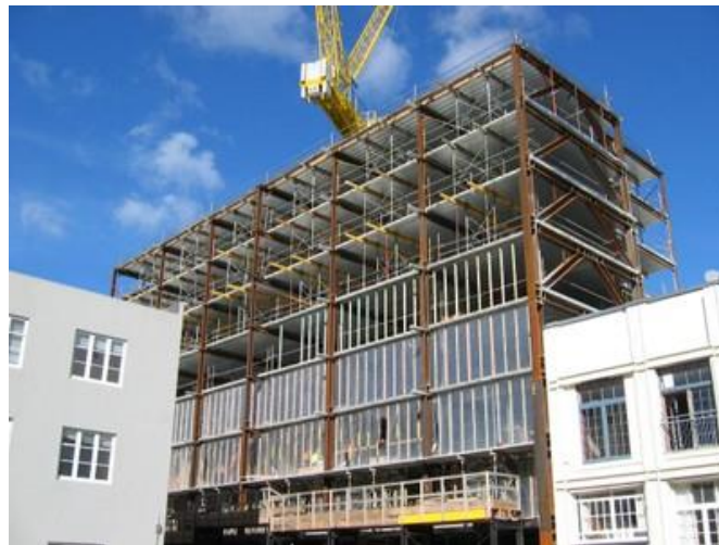
Fig. 2- 35. Eccentrically braced steel frame under construction, New Zealand (A. Charleson) [65]
