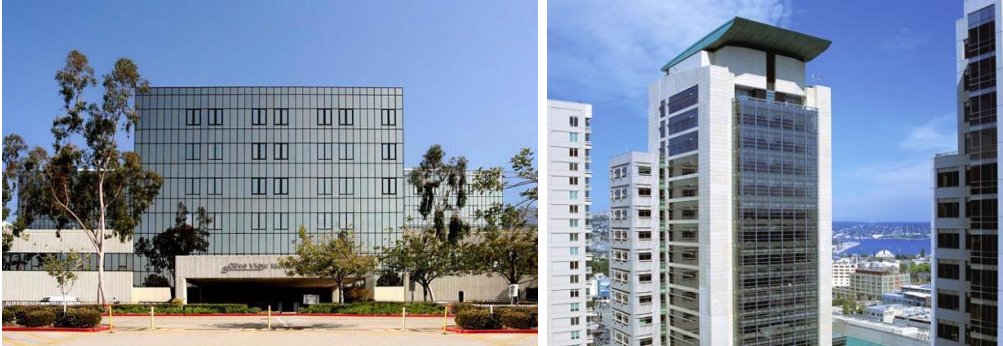
Fig. 2-31. SPSW buildings in USA: Olive View Hospital in Sylmar [61], California and US Federal Courthouse in Seattle [62]
