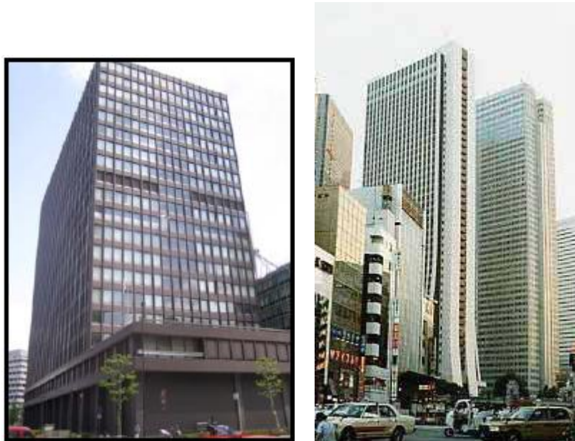
Fig. 2-32. SPSW buildings in Japan: Nippon Steel Building in Tokyo and Shinjuku Nomura Building [62]
