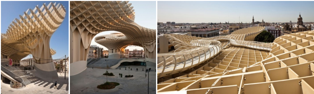
Fig. 5.3 Metropol Parasol - arh. Jurgen Mayer, Sevilla, Spania, 2011 162
