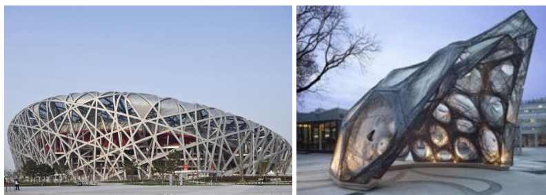
Fig. 4.26 (a) Jesere uniformă, Stadion olimpic- arh. Herzog& de Meuron, Beijing, China, 2008 122 ; (b) Jesere neuniformă, Pavilion experimental - arh. ICD-ITKE University of Stuttgart, Stuttgart, Germania, 2013 123
