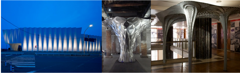
Fig. 5.28 (a) Pleats.M - arh. Hironaka Ogawa & Associates, Saitama, Japonia, 2012 199 ; (b) Arum - arh. Zaha Hadid Architects, Venetia, Italia, 2012 200 ; (c) ShellLace Structure - arh. Tonkin Liu, Londra, UK, 2014 201
