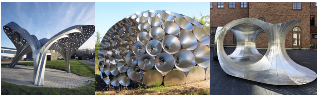
Fig. 5.8 Structuri autoportante din coli de oțel (a) Rainbow gate - arh. Tonkin Liu, Burnley, UK, 2012 166 ; (b) Shadow Pavilion- arh. PLY Architecture, Michigan, USA, 2009 167 ; (c) The Archipelago Pavilion - arh. Chalmers University of Technology, Copenhaga, Danemarca, 2012 168
