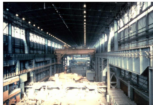
Figure 2-52 A steel mill in Bagnoli (Naples) (Mazzolani) [159] by courtesy of F.M. Mazzolani
