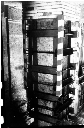
Figure 2-18 Consolidation of a masonry column (Mazzolani) [159] by courtesy of F.M. Mazzolani
