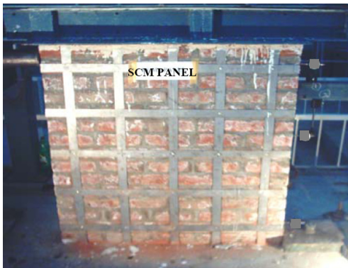
(a) Wall strengthened with steel mesh
