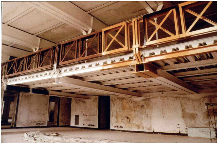
Figure 2-57 Example of insertion (Genoa, Italy) (Mazzolani) [159] by courtesy of F.M. Mazzolani
