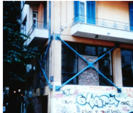
Figure 2-42 Building in Thessaloniki (Greece) (Mazzolani) [159] by courtesy of F.M. Mazzolani
