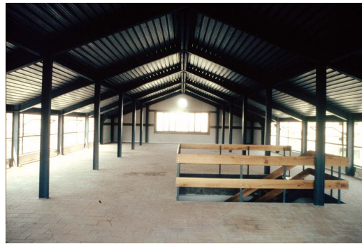
Figure 2-68 New spaces created in penthouse (Mazzolani) [159] by courtesy of F.M. Mazzolani
