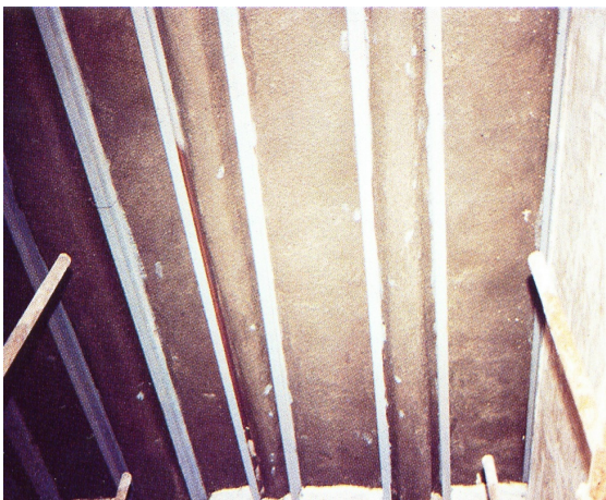
Figure 2-29 Example of intervention on a wooden floor (Mazzolani) [159]
