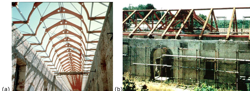
(a) (b) Figure 2-59 Examples of weight reduction by roof replacement (a. The Rivoli Museum , Torino, Italia; b. Mongiana Factory, Italia) (Mazzolani) [159] by courtesy of F.M. Mazzolani
