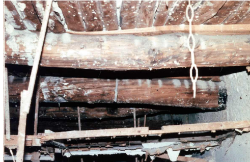
Figure 2-15. Old wooden floor (Mazzolani) [159] by courtesy of F.M. Mazzolani
