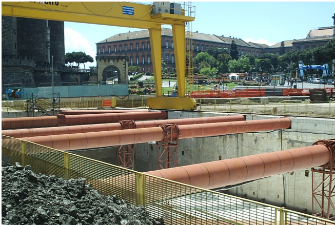
Figure 2-13 Naples underground station (Mazzolani) [159] by courtesy of F.M. Mazzolani
