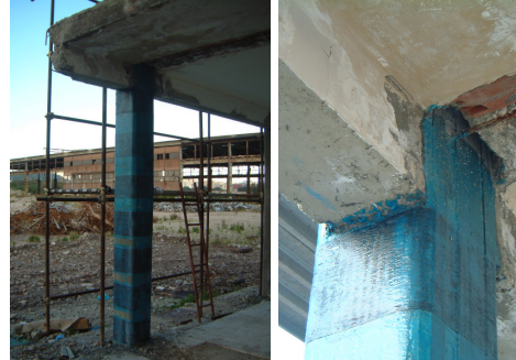
Figure 2-26 Repairing intervention on a r.c. column using CFRP (Mazzolani) [159]
