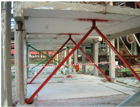
Figure 2-43 Reinforced concrete structure consolidated with EBF (Mazzolani) [159] by courtesy of F.M. Mazzolani
