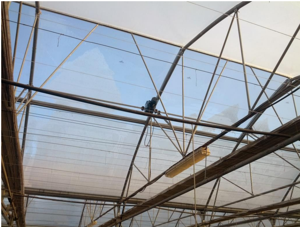
Fig. 2.10. Inside view of the greenhouse roof
