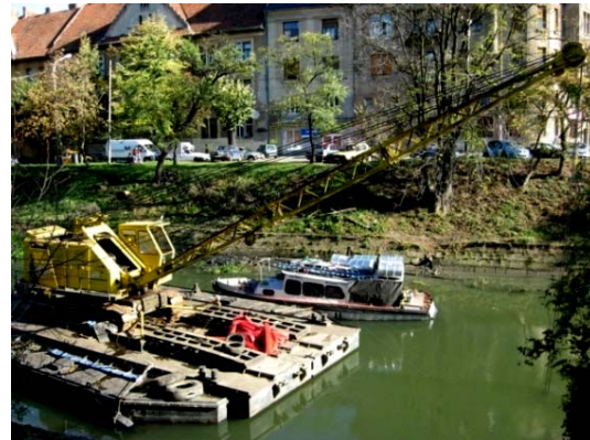
Figure 8. Dredging the Bega Channel
