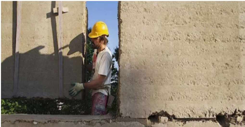
Fig. 236. Montarea panourilor prefabricate, sursă: © https://www.architectural-review.com/buildings/earth/ricola-herb-centre-in-switzerland-by-herzog-and-de-meuron-with-martin-rauch , ultima accesare: 12.2020;
