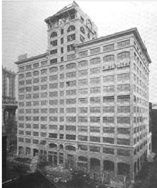
b) Clocktower Building, 1914 [3]
