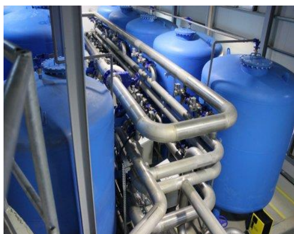
Figure 3. Proposed Treatment Plant - sand filters + GAC filters
