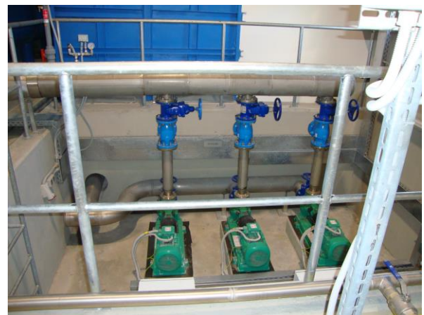
Figure 2. Treatment Plant proposed - influent pumps / wash filters
