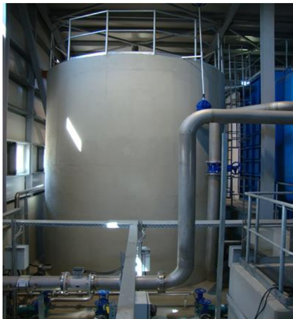
Figure 4. Sequential Decanter for water washing treatment
