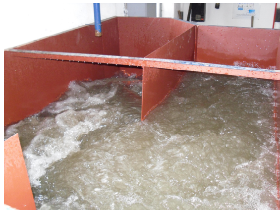
Figura 3.2. Camera de amestec
