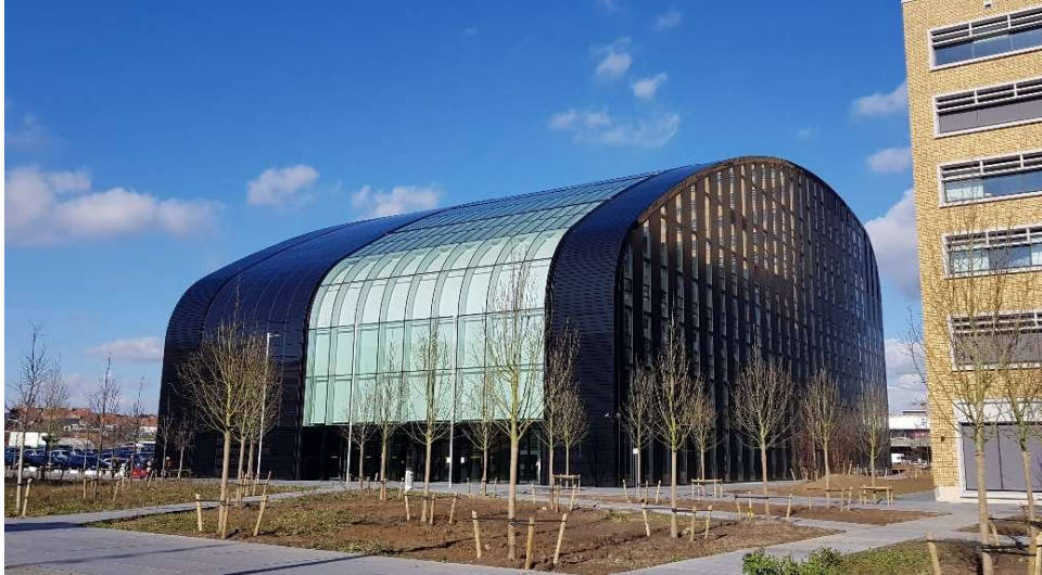
Fig. 1-6. Brussels Environment Building [27]
