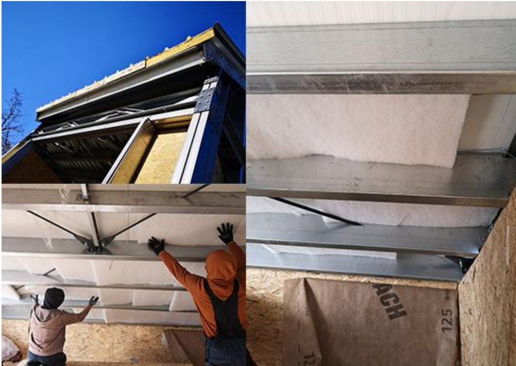
Figure 4.18. Steel structure / roof component assembly
