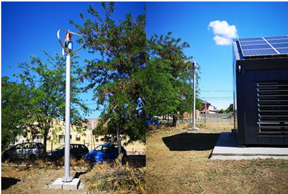
Figure 4.31. On-site wind turbine
