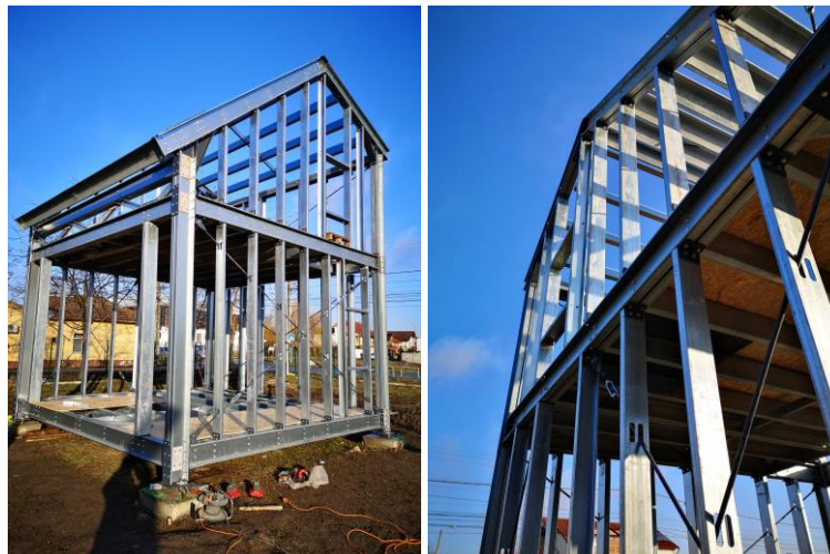
Figure 4.14. Steel structure assembly
