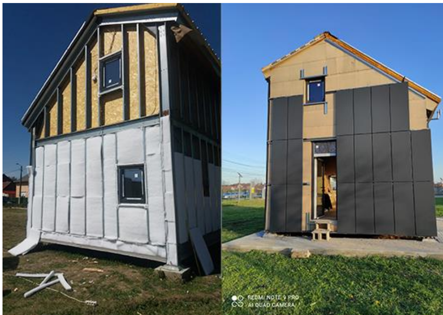
Figure 4.22. Wall element assembly.
