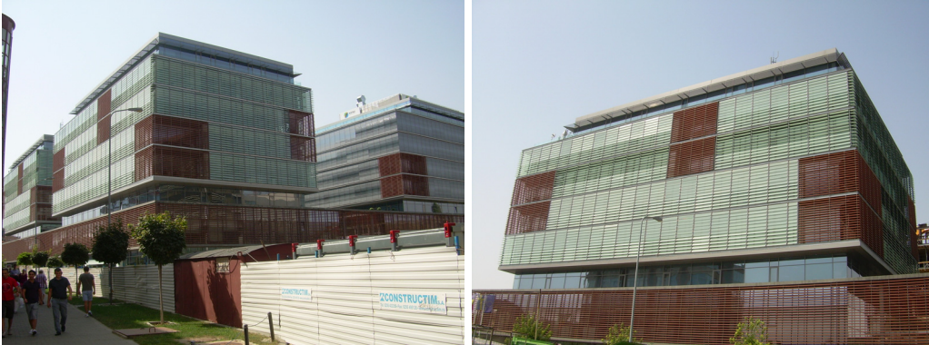
Fig. 7.5. City Business Centre P-ța 700, Timișoara
