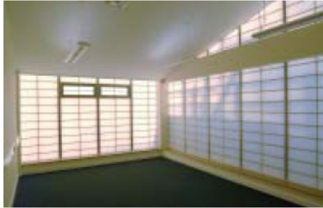
Fig.3.81. Jersey General Hospital
