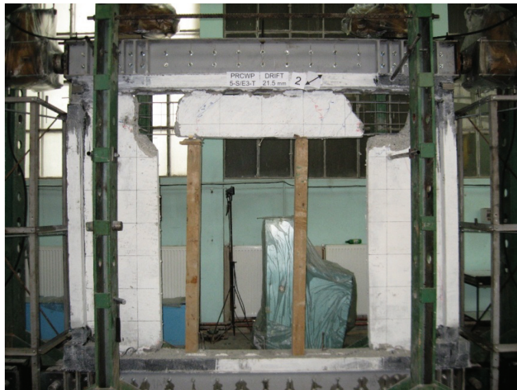
Figure E.53 Failure detail PRCWP 5-S/E3-T: general view after the crushed concrete was removed
