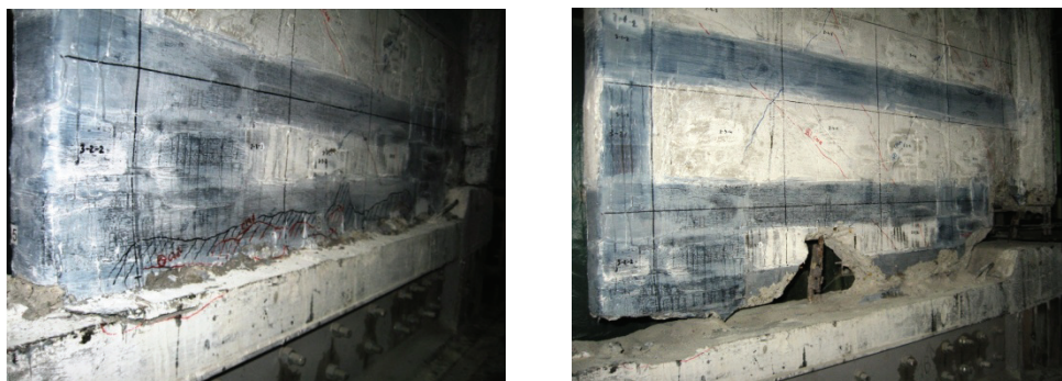
Figure E.91 Failure detail PRCWP 4-S/E1-R/T: the base of pier#2 at failure and after the crushed concrete was removed (obs. grids 3-2, 2-3, 2-2)
