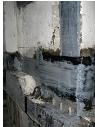
Figure B.6 FRP layout detail at the base anchorage of PRCWP 5-S/E3-T/R
