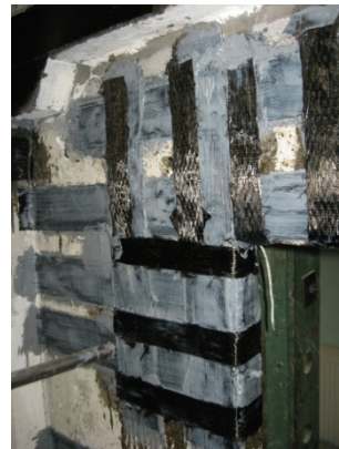
Figure B.5 FRP layout detail at the pier-to-beam connection of PRCWP 3-S/E1-T/R
