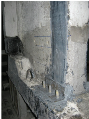
Figure B.6 FRP layout detail at the base anchorage of PRCWP 5-S/E3-T/R
