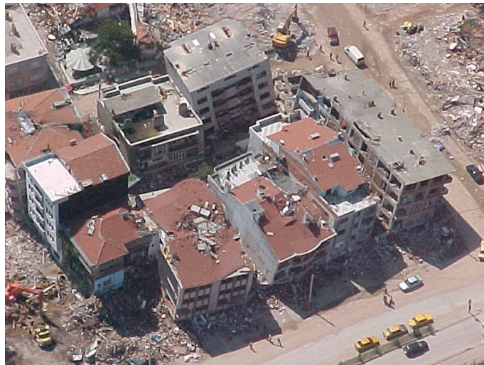
Figure 2.1 Buildings damaged by the 1999 Kocaeli, Turkey earthquake (EERI, [4])
