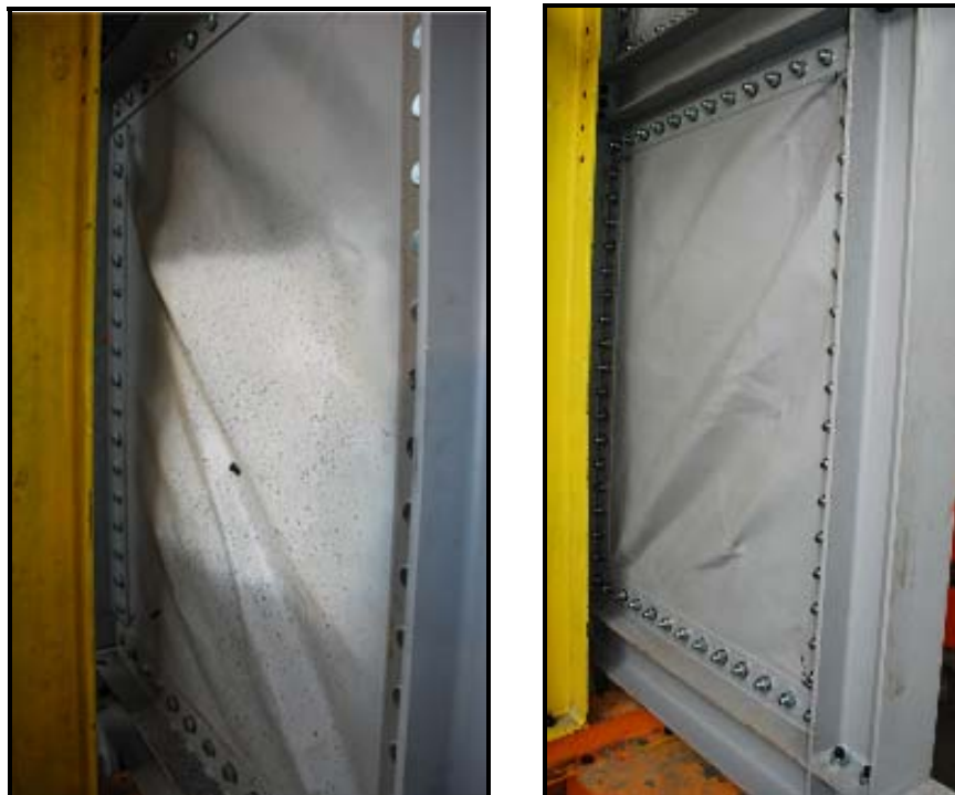
Figure 28 - Final stage of plate (both sides)
