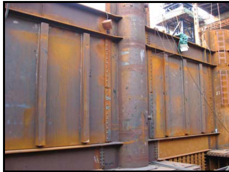
Figure 2-44 - Buckling Restrained SPSWs
