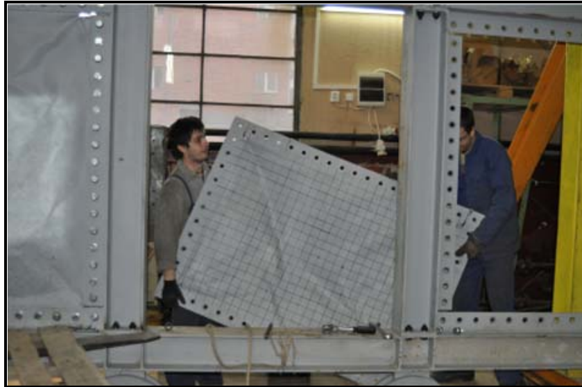
Figure 37 - Infill plate dismantling
