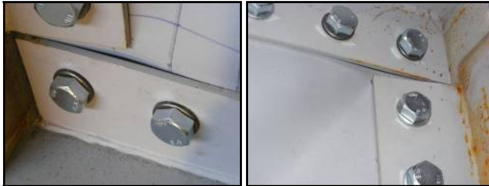
Figure 35 - Details of infill plates corners
