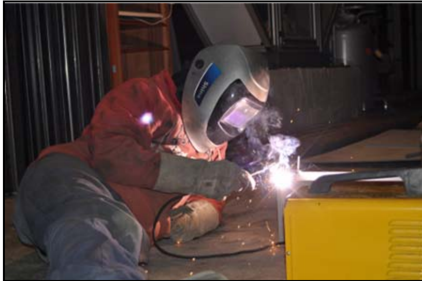
Figure 10 – Measuring devices support welding
