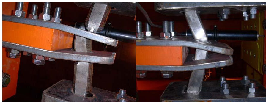
Figure 2.24 Deformed pin connections after test [19]
