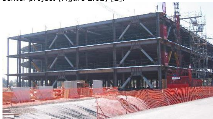
Figure 2.62 Kaiser Santa Clara under construction [2]
