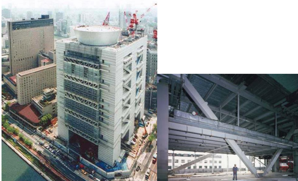
Figure 2.56 Osaka International Convention Center ("damage tolerant" structural design, $420 million project, completed in 1999, 721000 s.f., 13+2 storeys, h=300 ft, 370 braces, largest 73 ft with P_y = 1200 kips) [26]
