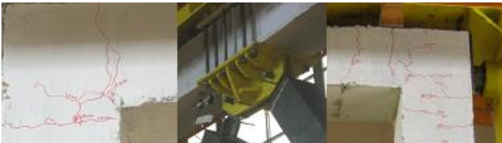
Figure 6.29 MRF+BRB under cyclic load – bending moment cracks
