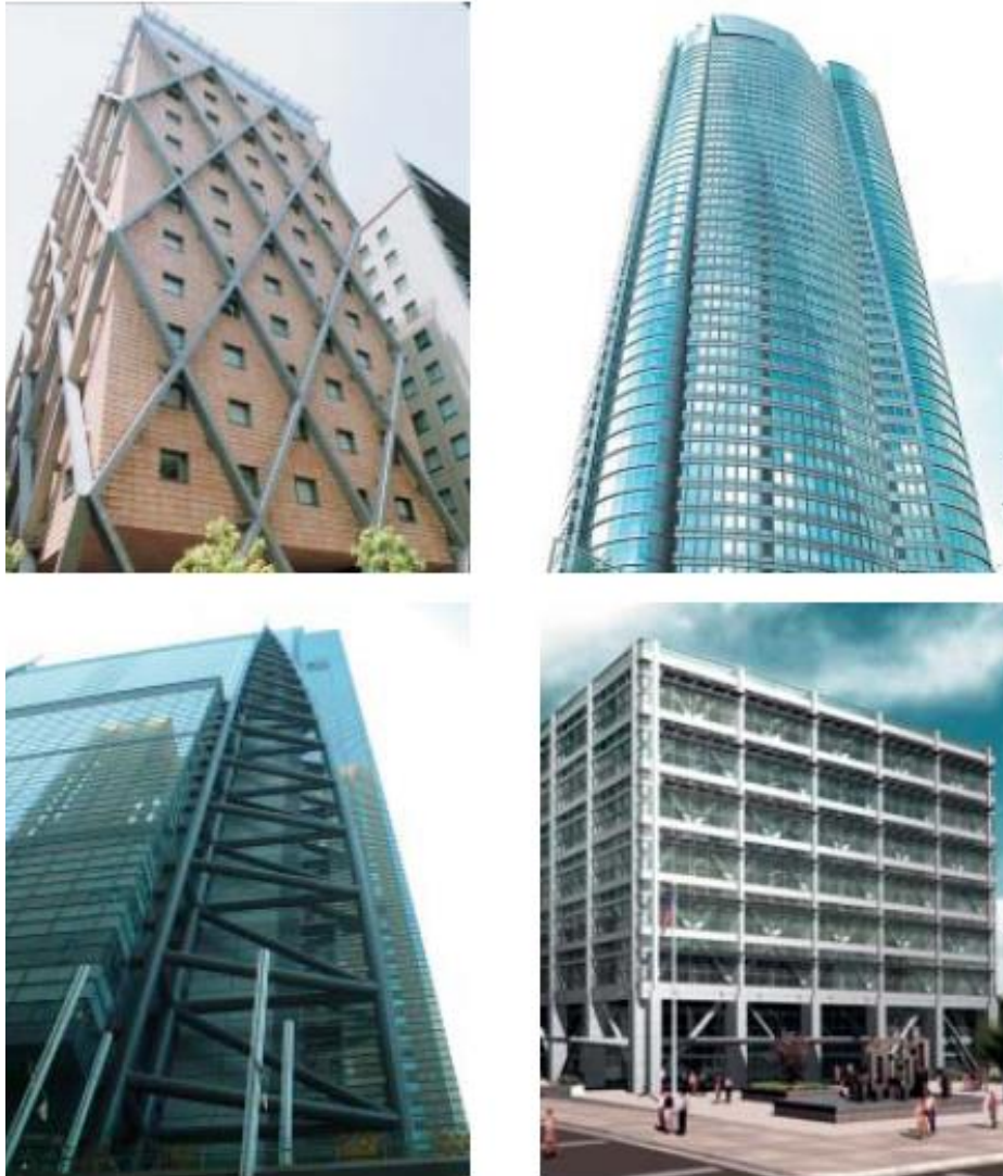
Figure 2.60 Exterior exposition system, rectangular tube type: (upper left) SANKYO New Tokyo Headquarter Building (Tokyo, 1997); Nippon Television Tower (Tokyo, 2003) (lower left); Roppongi Hills (Tokyo, 2002); Seismic reinforcement of US Federal Government Building (Salt Lake, U.S., 2001) [4]
