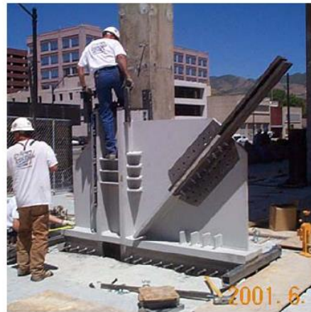
Brace connection assembly ready for installation at Grid Q'-2'
