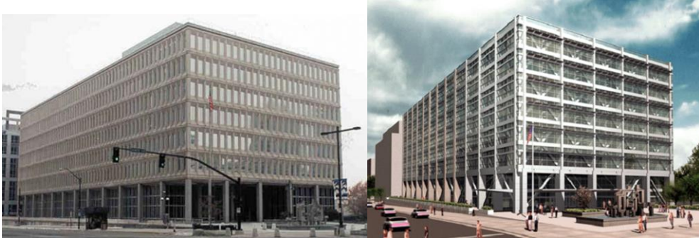
Figure 2.66 Wallace F. Bennett Federal Building Before Retrofitting and After Retrofitting [42]
