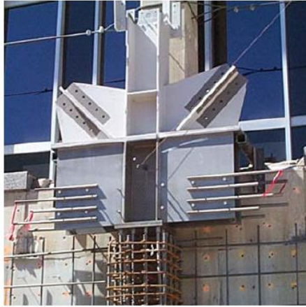
Shear transfer assembly and brace connection during construction
