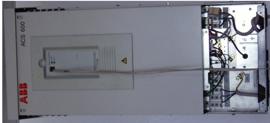
Fig. 7.2. Bidirectional three phase inverter ACS600
