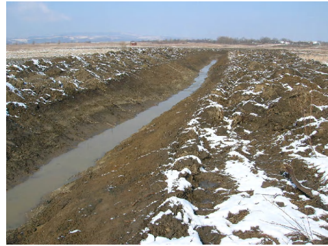
Photo 12 – Drainage channels CCS42 during execution (2008)
