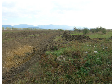
Photo 14 – Secondary drainage channel CT40321 (2008)
