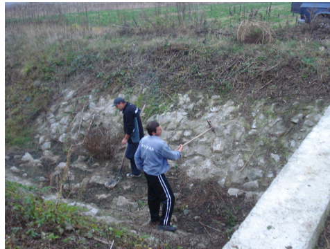
Photo 8 - Maintenance works on pipes at drainage channel CCS43 (2010)
