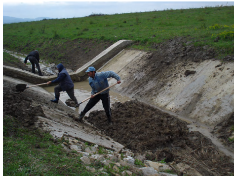
Photo 9 – Drainage channel CT4032 Cleaning works at the threshold drops (2009)
