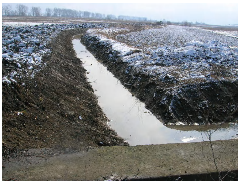
Photo 13 – Secondary drainage channel CT425 (2008)
