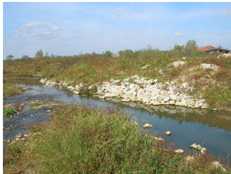
Photo 20 – Lisava Valley Consolidation with rough stone at the junction with cu Oravita Valley (2010) Oravita Valley and three Lisava Valley;
