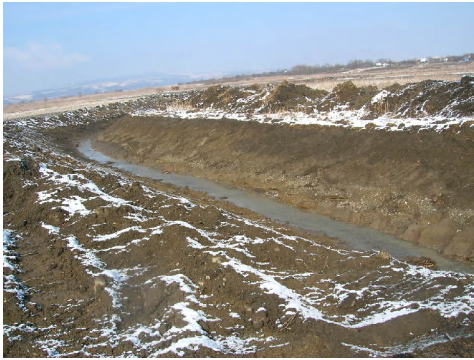
Photo 11 – Drainage channel CCS43 during execution (2008)
