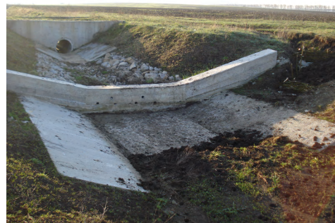
Photo 10 – Pipe culvert DN800 and threshold drop at drainage channel CS410 (2009)
