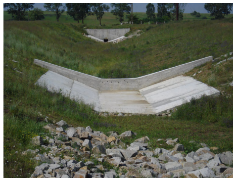
Photo 17 – Threshold drops, pipe DN1000 and consolidation at the junction with Lisava Valley of drainage channel CP41 (2010)
