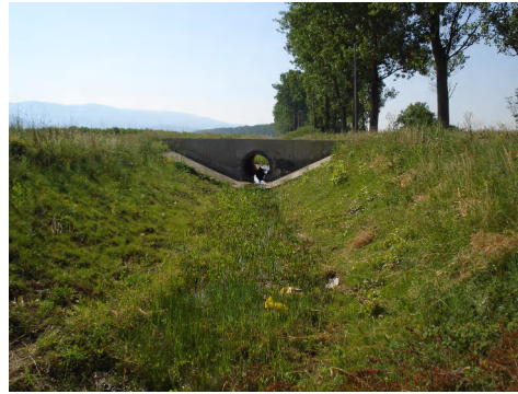
Photo 16 – Pipe DN1200 on drainage channel CP41 (2010)
