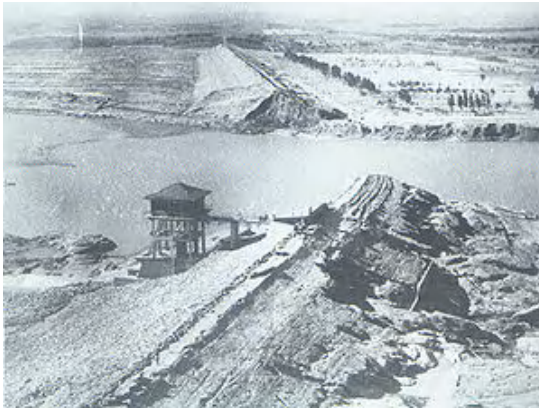
Fig.3 Banqiao Dam after the break.
