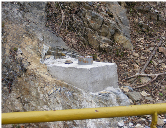
Fig. 5 Stationary height mark at Petrimanu dam
