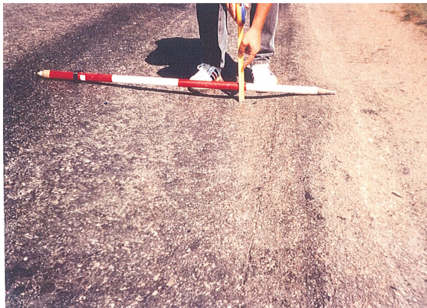
Fig. 2. Cracking with settlement
