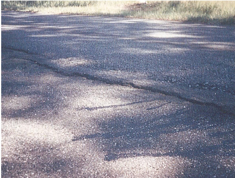
Fig. 2. Cracking with settlement
