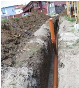
g) Ground-air heat exchanger
