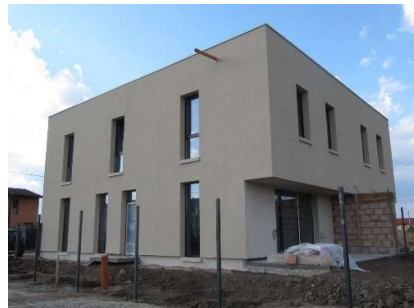
h) South-West and South-East facades
