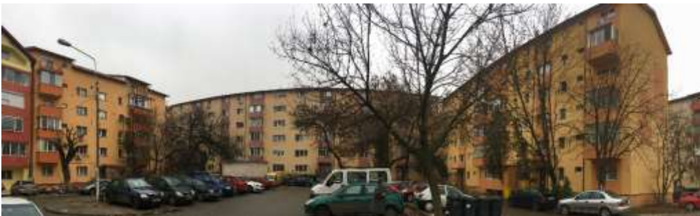
Figure 2-14 – Panoramic view of precast buildings neighbourhood
