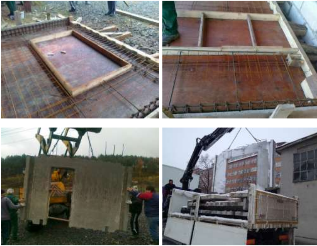
Figure 3-3 – Construction of the specimens (Stei)
