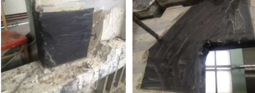
Figure 3-16 – NSM-CFRP combined with EBR-CFRP strengthening process
