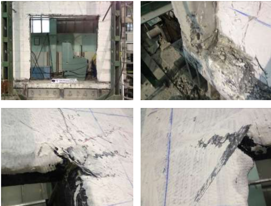
Figure 4-6 – Failure details of PRCWP 13-S-E3-RT
