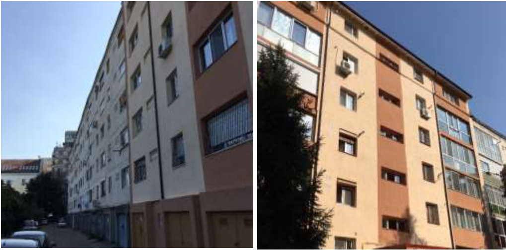
Figure 2-12 – P+4 project type 770-81 precast building, original and with attic added later
