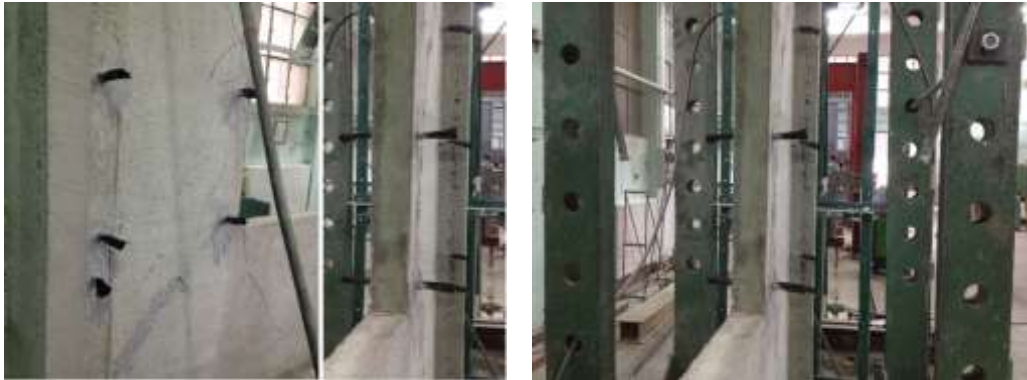
Figure 3-19 – Anchorages for the EBR CFRP system
