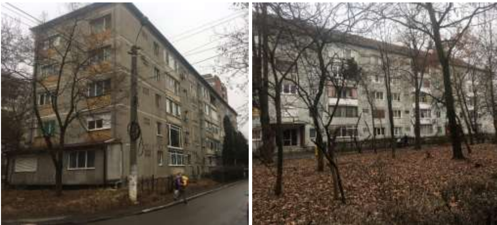
Figure 2-13 – P+4 typical precast apartment buildings
