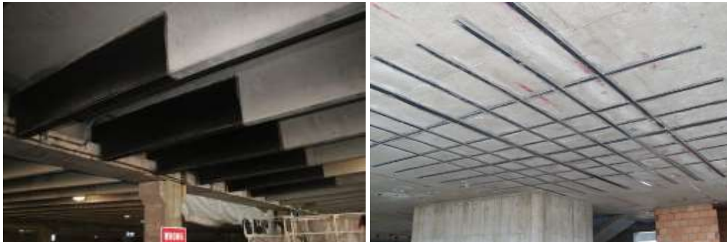
Figure 2-24 – EBR system for mesh and laminates [137, 138]
