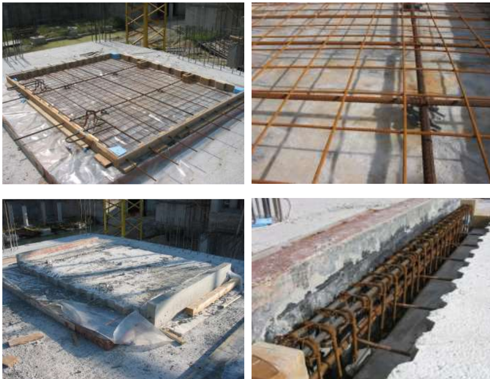
Figure 3-2 – Construction of the specimens (Timisoara)
