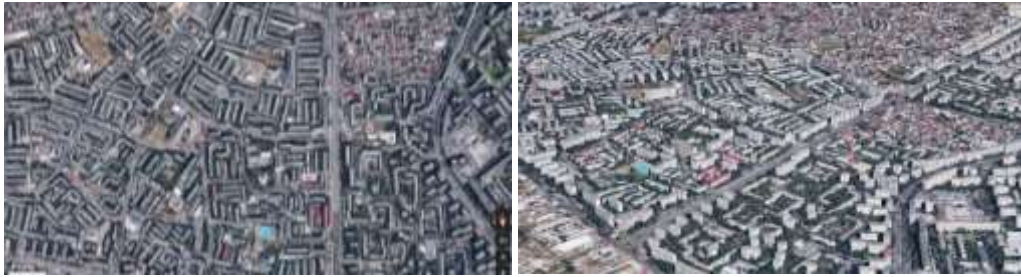
Figure 2-15 – Precast buildings neighbourhood in Bucharest [53]
