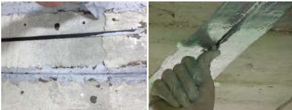
Figure 2-25 – NSM system for CFRP laminates [139]
