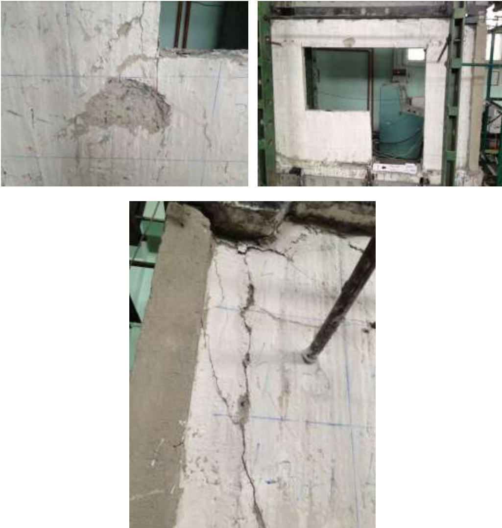
Figure 4-1 – Failure details of PRCWP 14-S-EL2-T
