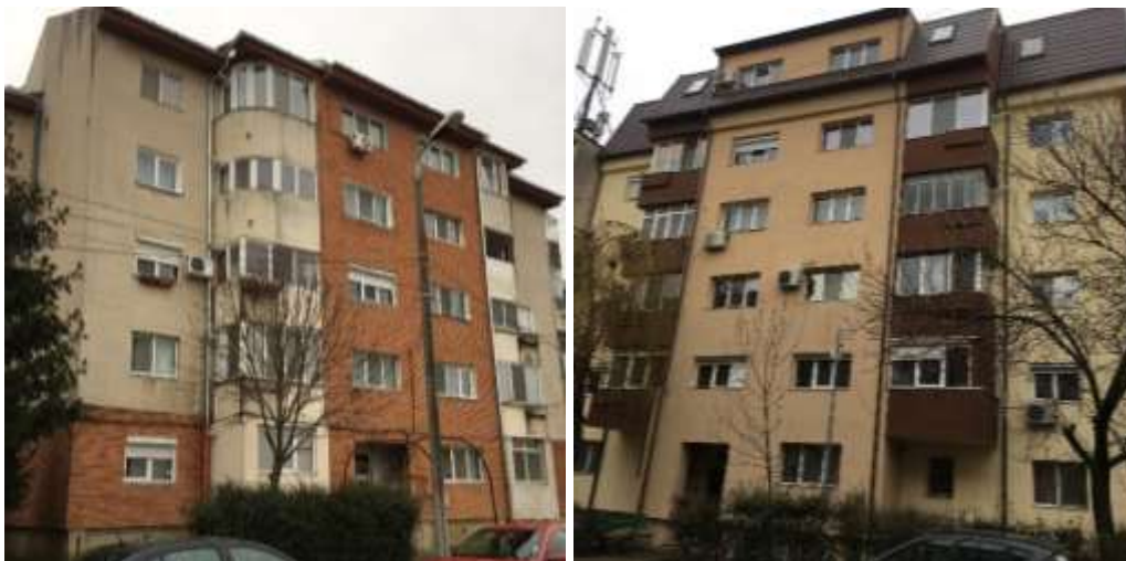
Figure 2-11 – P+4 project type 770-81 precast building, original and with attic added later
