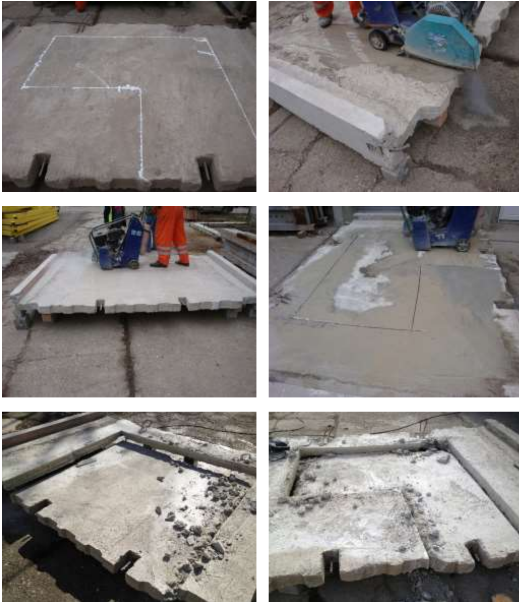
Figure 3-4 – Opening cut-out procedure
