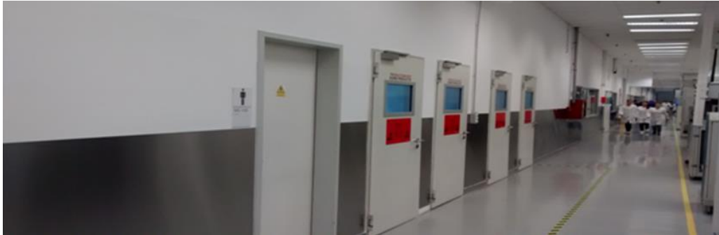
Figure 2.42. After wall plating with stainless steel
