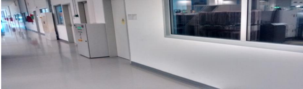
Figure 2.41. Before wall plating with stainless steel
