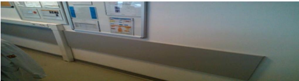
Figure 2.48. Meeting room appearance (after)
