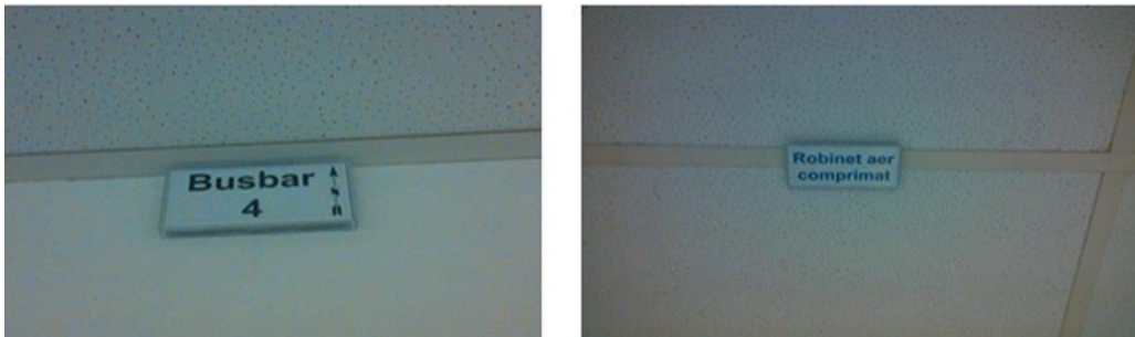
Figure 2.43. After electrical circuit and HVAV labeling
