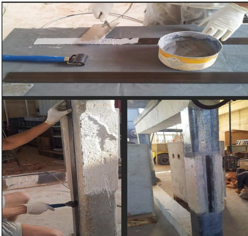
Fig. 4.31. Aplicarea lamelelor Sika Carbodur S512
