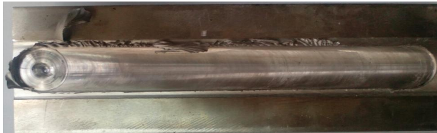
Figure 2—26 The face of weld metal of the second T-joint
