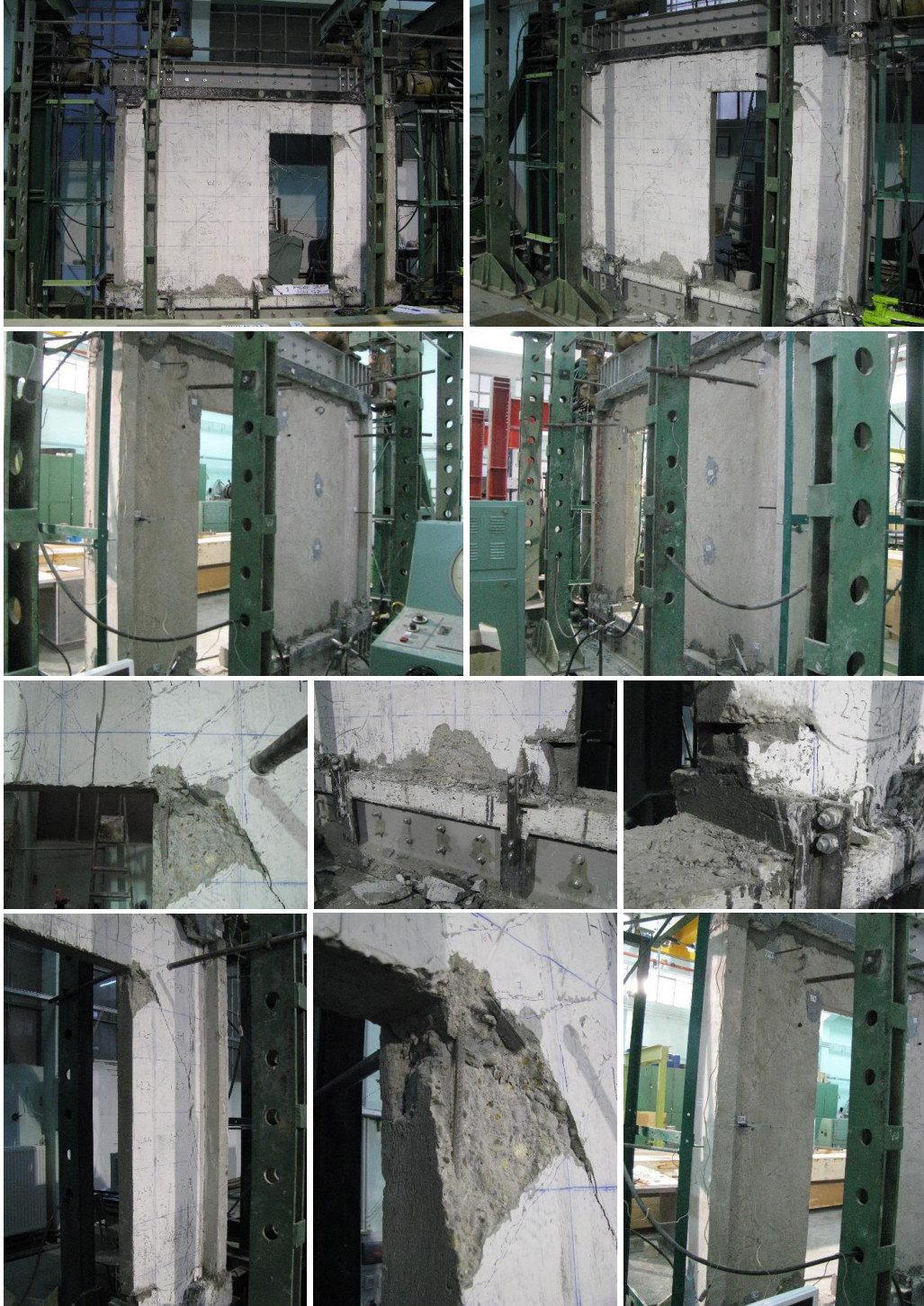
Figure 2.25 – PRCWP (12-E1-T) failure details [108-109]
