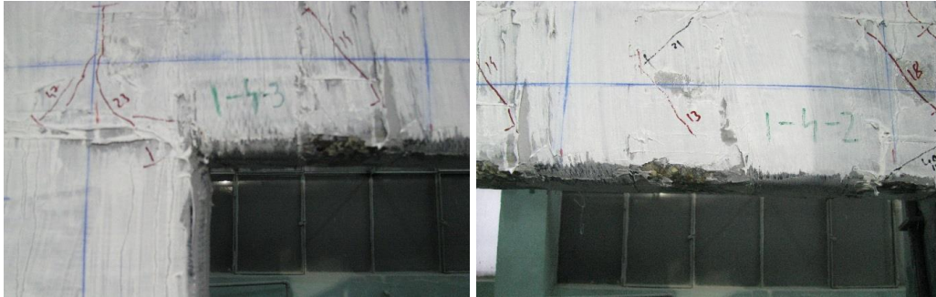
Figure 3.6 - Failure details of the PRCWP (12-E1-T/R) specimen [109, 120]
