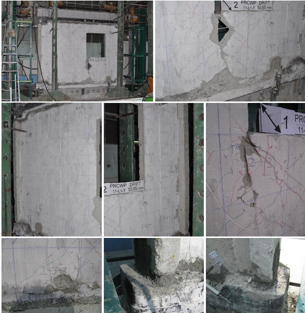
Figure 2.24 – PRCWP (11-L1-T) failure details [108-109, 113-114, 116]
