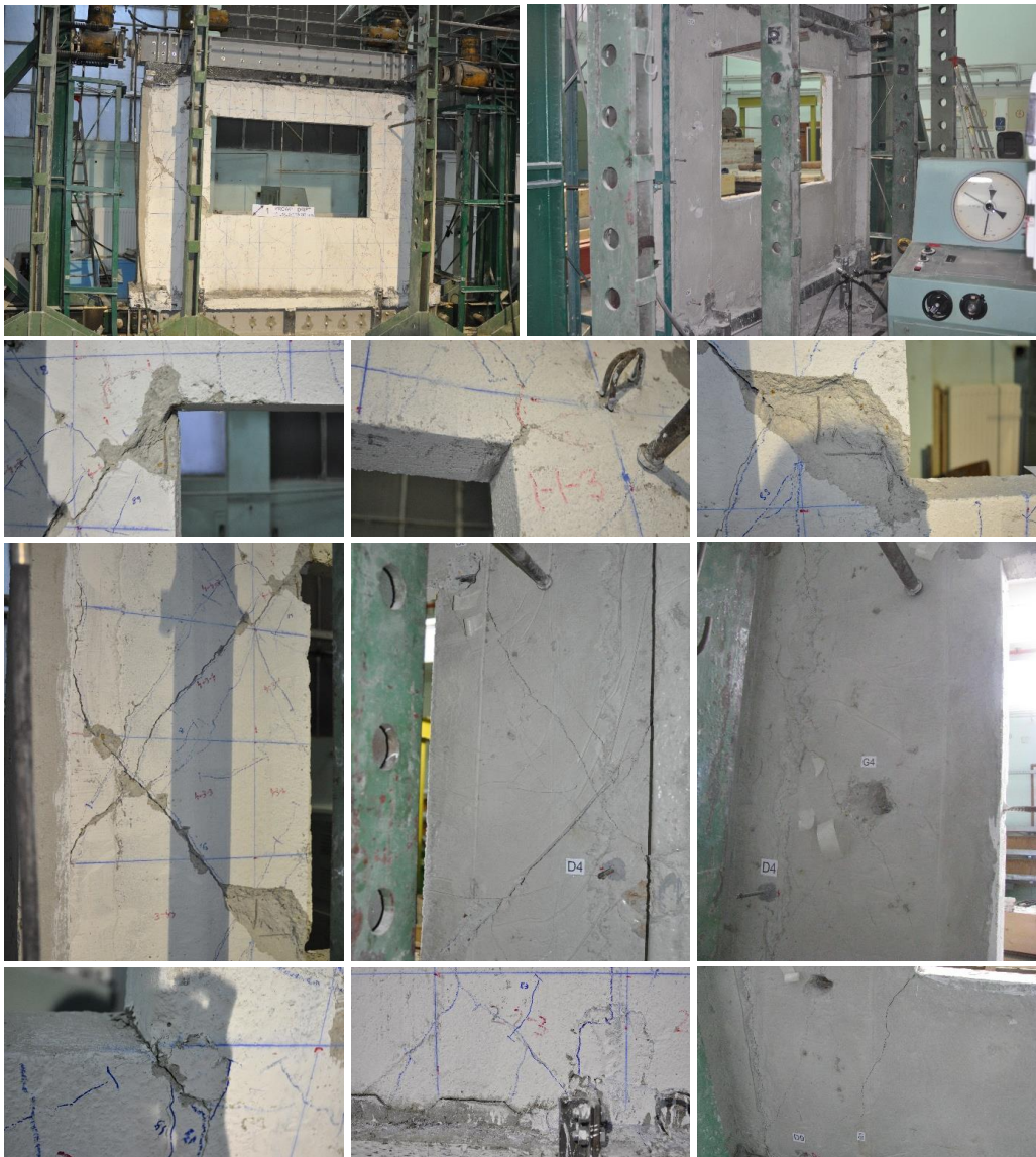
Figure 2.23 – PRCWP (10-L1/L3-T) failure details [108-109, 111-112, 116]
