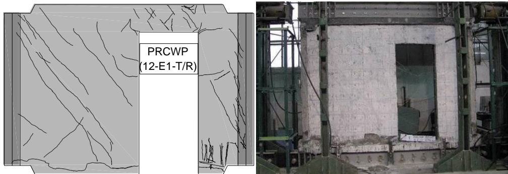
Figure 3.61 The final cracking pattern of the tested specimens
