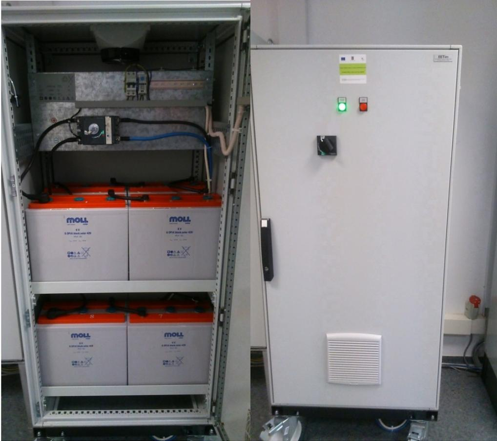
Fig. 4.3. A 50 V, 400 Ah battery stack emulating a storage system
