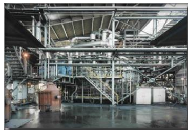
Figura 3.26. Procedeele Fastmet, Uzina Kobe Steel Kakogawa Works
