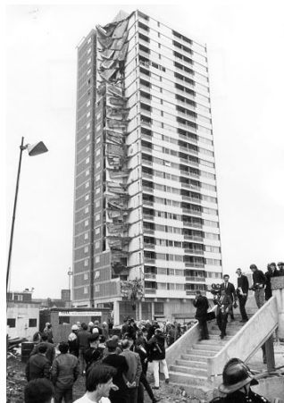
Figure 2.1 Ronan Point Collapse, 1968, London, UK [16]
