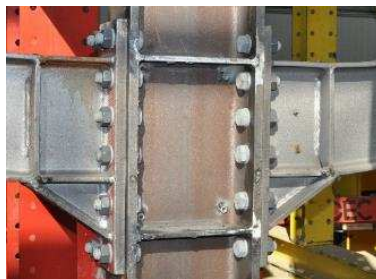
d) central column joint after the test
