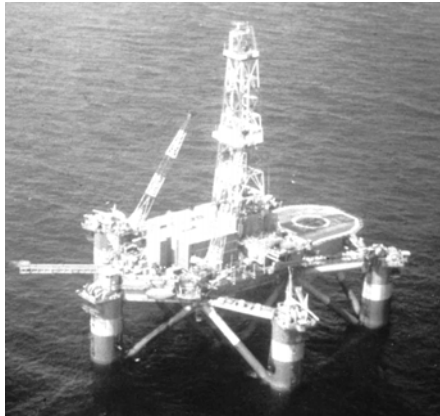
Fig. 1.9. Alexander L Kielland oil platform
