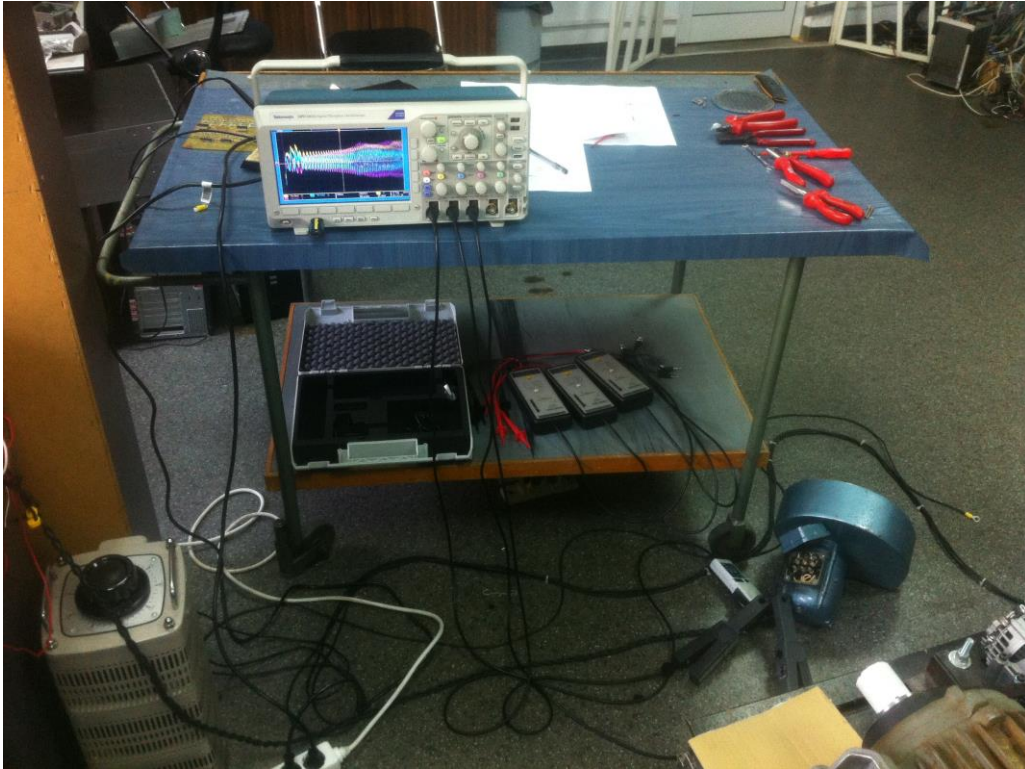
Figure 5.29 Auto-transformer for charging the Z-source network, induction machine and the measurement system.
