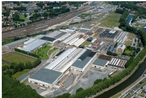
Figure 3.4. Bombardier transportation Belgium production site
