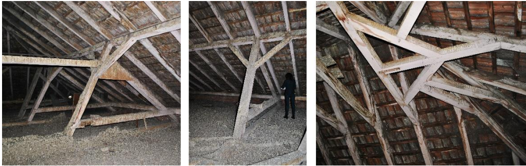
Fig. 5.8 Early 19 th century roof structure type
