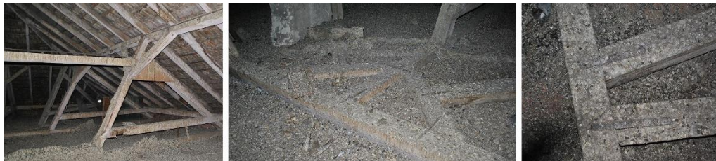
Fig. 2.35 Pigeon droppings deposit
