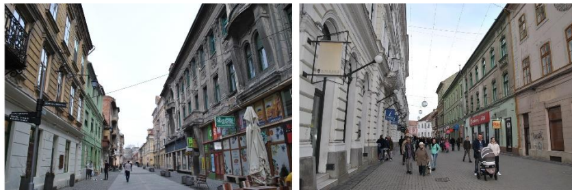
Fig. 2.12 Roof structures with no urban value placed along narrow streets
