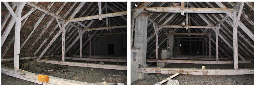
Fig. 5.9 I.C. Bratianu high school – late 19 th century roof structure (right side)
