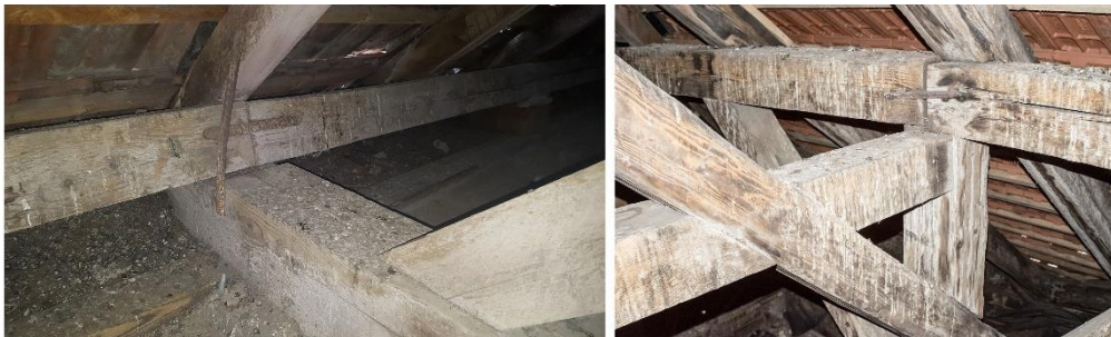
Fig. 2.33 Scarf joint with steel fastener
