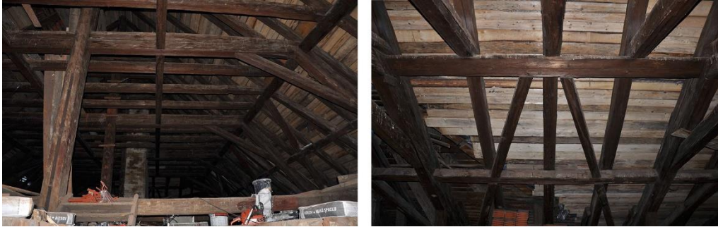
Fig. 5.7 Union square 18 th century roof structure
