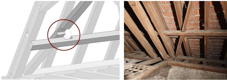
Fig. 2.32 Lap joint
