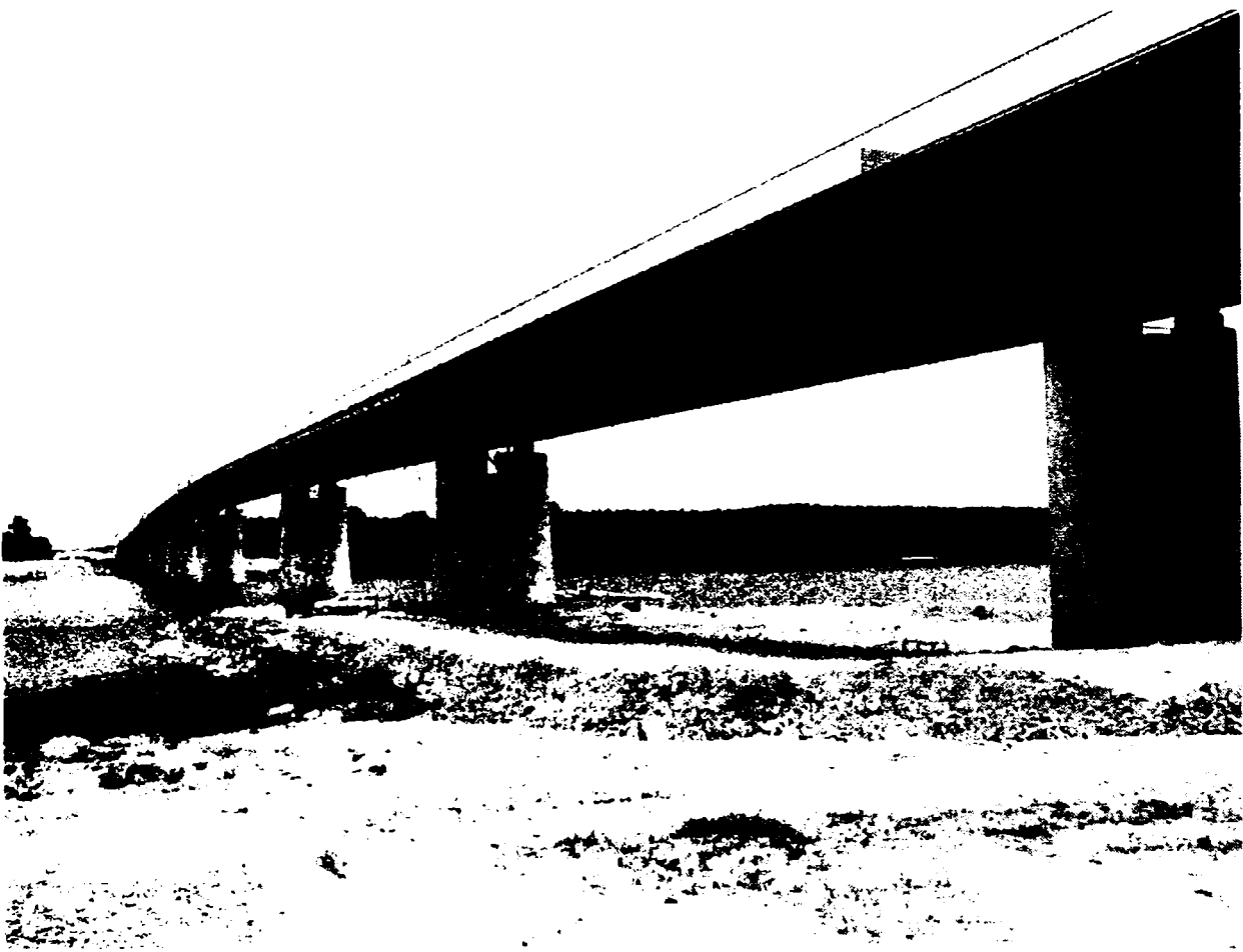
Fig. 2.56. View of the full bridge
