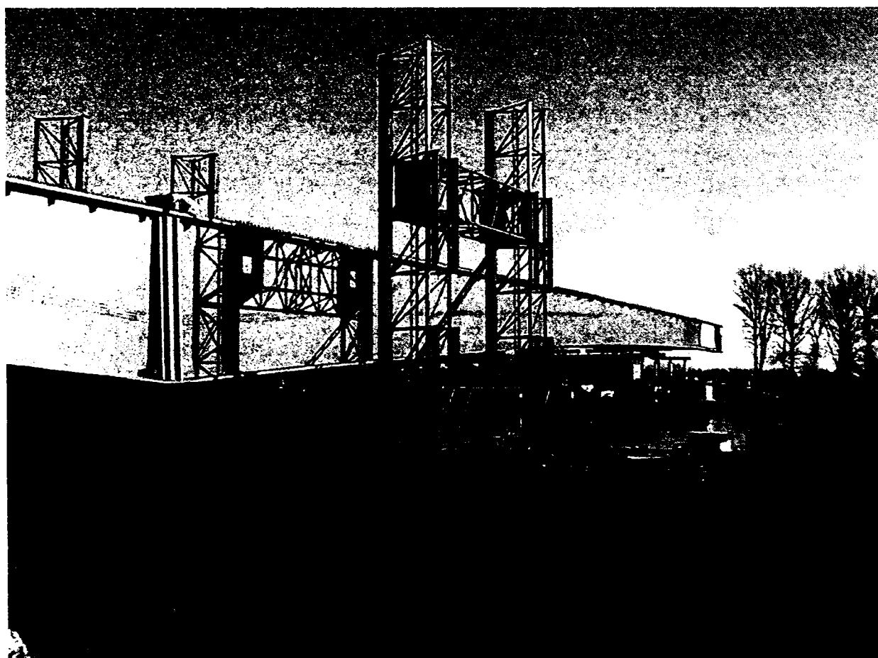
Fig. 2.35. Putting the bridge in place
