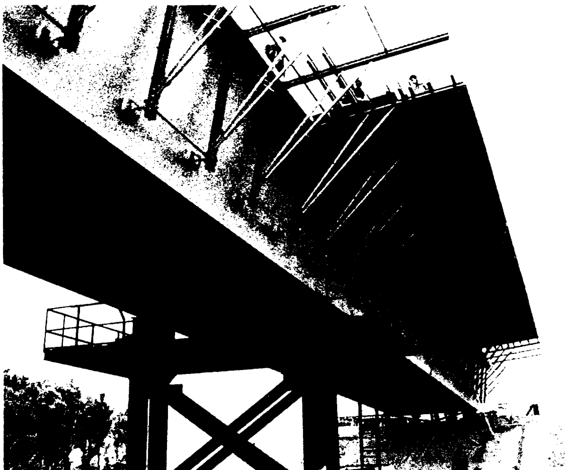
Fig. 2.53. View of the propped box girder
