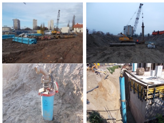
Figure 10. Photos during the boreholes installation
