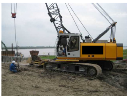
Figure 3. Pumps installation and commissioning
