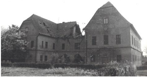
(a) - North façade
