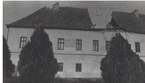
(b) - South façade
