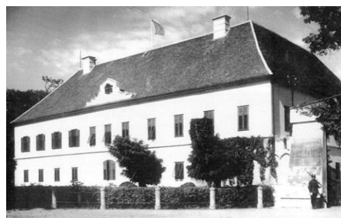
(b) – South façade, 1936
