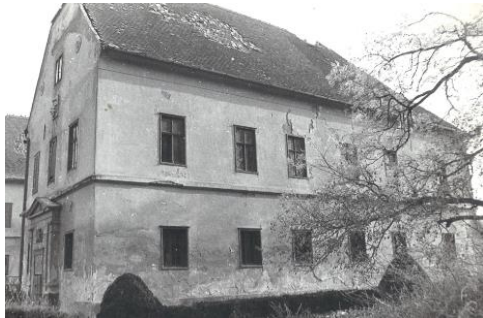
(c) – North-West façade
