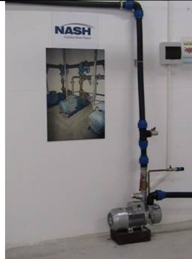
Fig.4.5 Pompa de vacuum tip NASH
