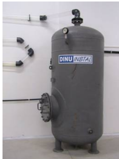
Fig. 4.3 Rezervor vacuum
