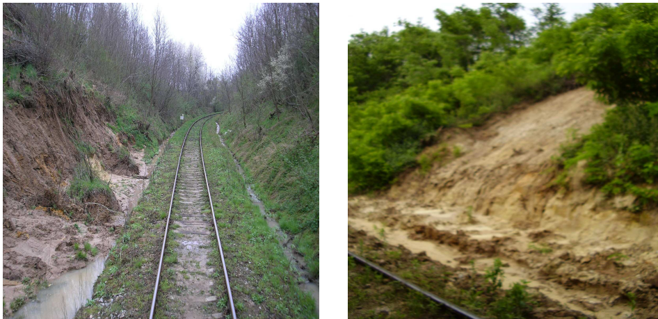
Fig.5.49 Alunecare taluz debleu linia 130 Berzovia - Oravița km.16+500 - km.16+700
