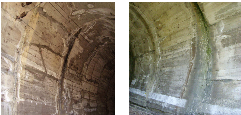
Fig.5.41 Detaliu interior tunel km.66+660 - km.67+277
