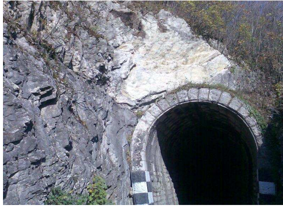
Fig.5.60 Portal intrare tunel km.19+673
