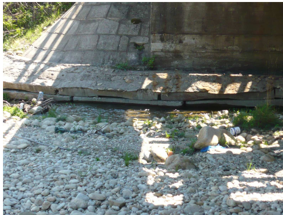
Fig.5.31 Consolidarea culee cu traverse de beton armat pod km.36+673 linia 116
