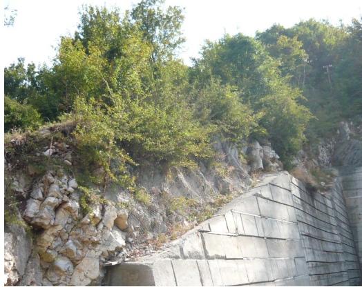
Fig.5.63 Prelungire aripă tunel km.25+356 - km.26+016
