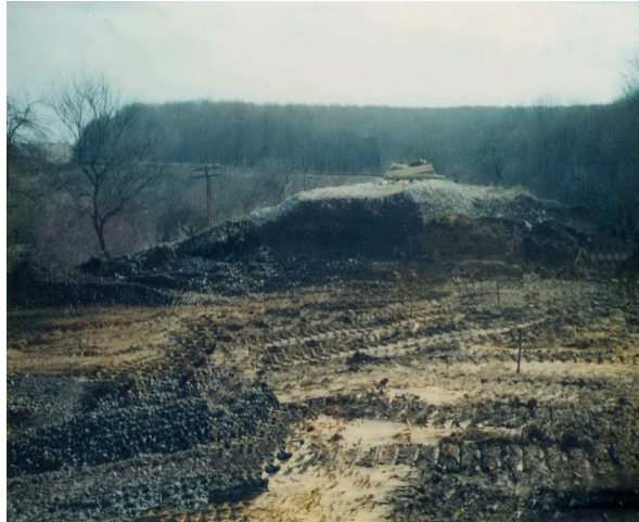
Fig.6.18 Refacere terasament km.25+315 ... km.25+435
