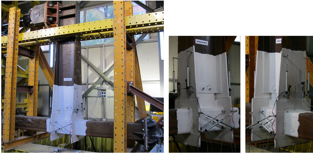
Fig. 5-81. S700-CP-R test assembly and connection zone – before test
