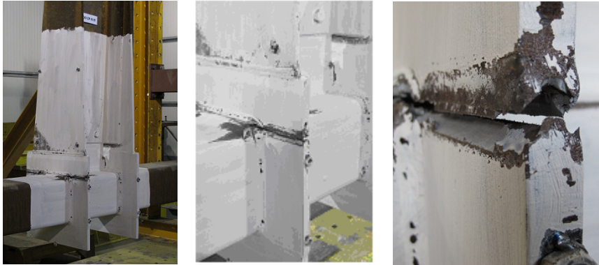
Fig. 5-104. Weld failure within S700-CP-R-M joint
