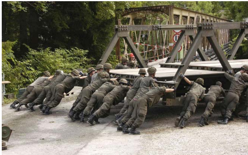
Figure 3.17 – Launching of a D-Bridge (Image courtesy of Austrian Armed Forces [21])
