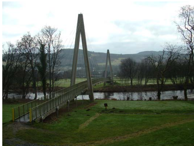
Figure 1.4 – All-FRP Aberfeldy Footbridge over the River Tay
