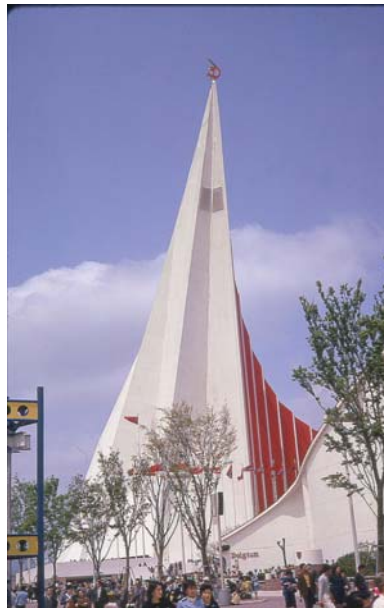
Figure 1.2 – Example of selection of FRP as structural material: pavilion of the USSR at the Osaka World Trade Fair Expo 1970 [76].
