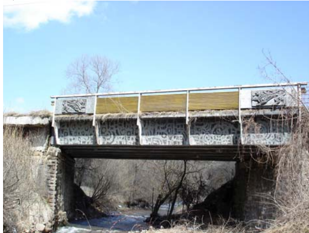
Figure 1.3 – Ginzi Highway GFRP- Bridge, Bulgaria
