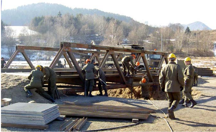
Figure 3.18 – Installation of a D-Bridge (Image courtesy of Austrian Armed Forces [21])
