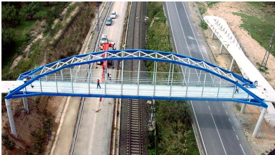
Figure 1.6 – The Lleida Bridge in Spain (Image courtesy of Fiberline Composites A/S [4])
