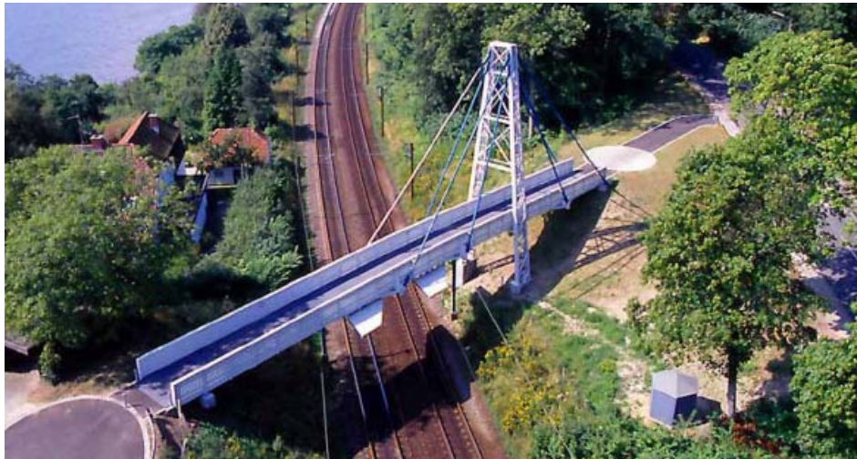
Figure 1.5 – The Fiberline Bridge in Kolding, Denmark (Image courtesy of Fiberline Composites A/S [4])
