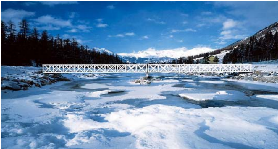
Figure 1.7 - The Pontresina Bridge, Switzerland (Image courtesy of Fiberline Composites A/S [4])
