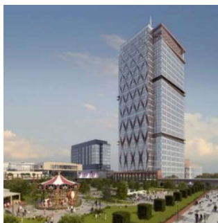
Figura 1.17. United Business Center 0, Timișoara
