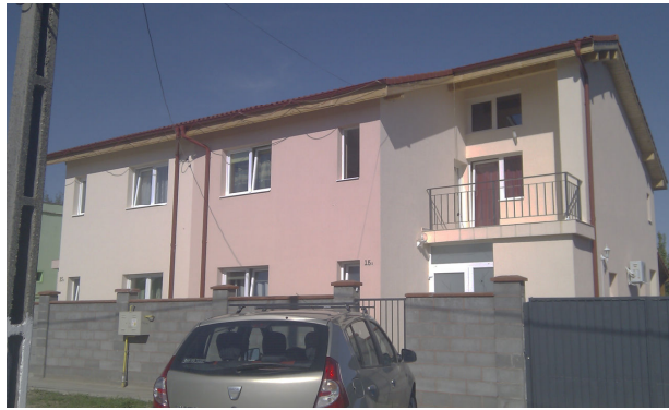
Figure 4.1. Front view of the studied building
