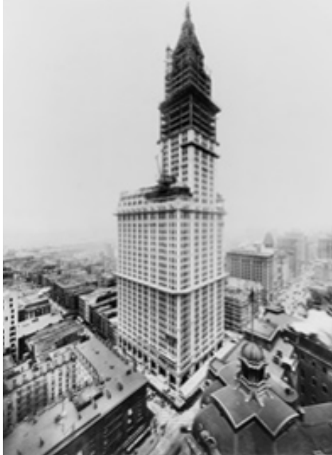
Figure 2.7 The Woolworth Building, New York http://www.ce.jhu.edu
