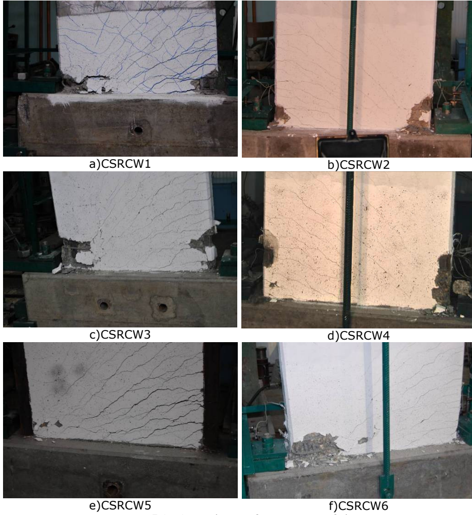
Figure 5.27 General view of specimens at failure
