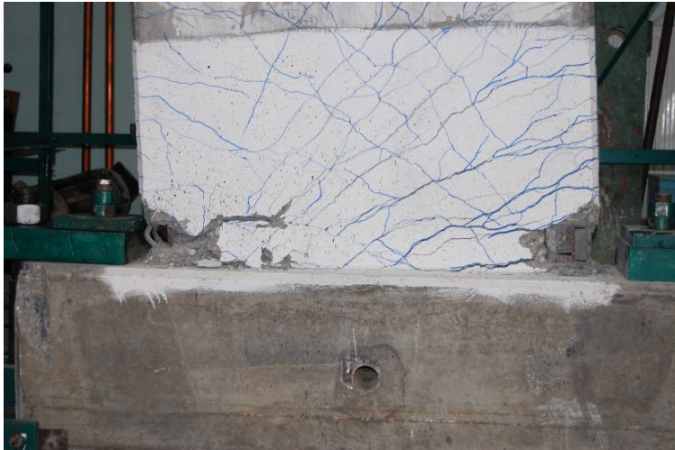
Figure B.1 Specimen CSRCW1 at failure
