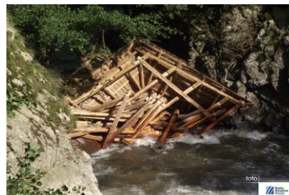
Figure 7. Other mill from Rudaria after the floods.
