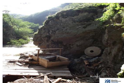
Figure 6. Mill from Rudaria after the floods.
