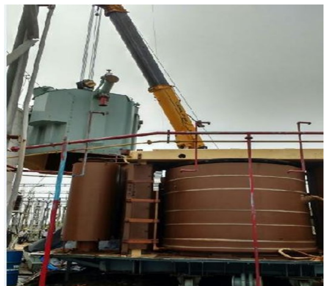
Fig. 11. Inspection of active part of transformer
