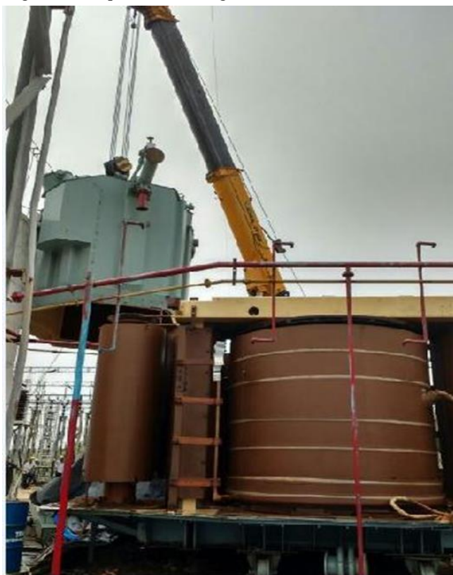
Fig. 3. Inspection of active part of transformer
