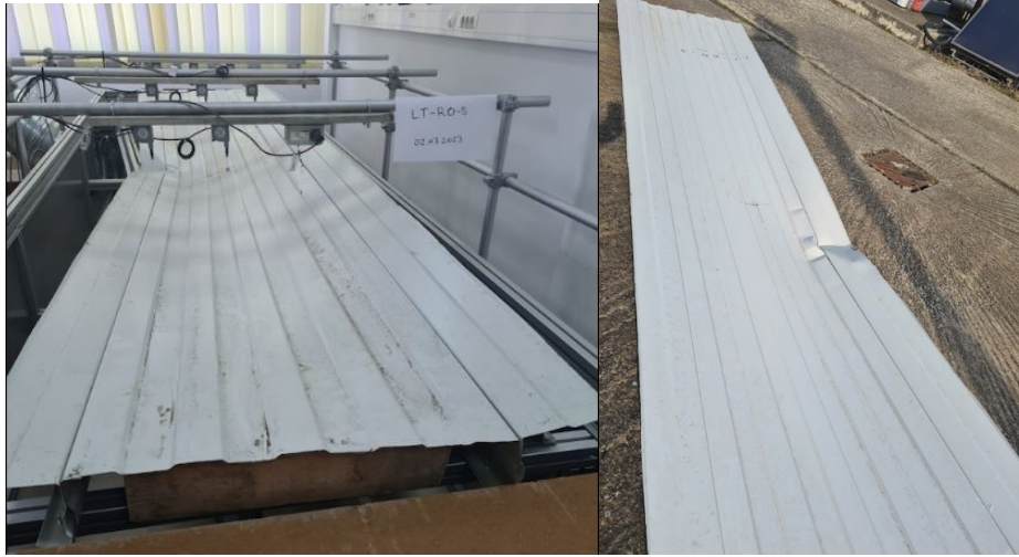
Figure 3.58 LT-RO-S specimen after failure: typical non-symmetric failure at mid-span
