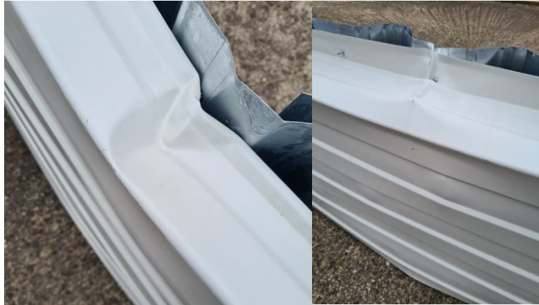
Figure 3.39 Detail of the failure zone on both sides of the liner tray: interaction between local+distortional buckling of the narrow flange and local+distortional buckling of the webs of restrained-opened liner trays
