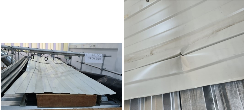
Figure 3.62 LT-RC-S specimen failure at mid-span
