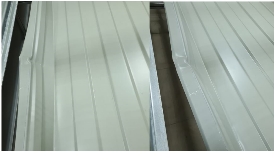
Figure 3.34 Detail of the failure zone; interaction between local buckling of the narrow flange and distortional buckling of the web
