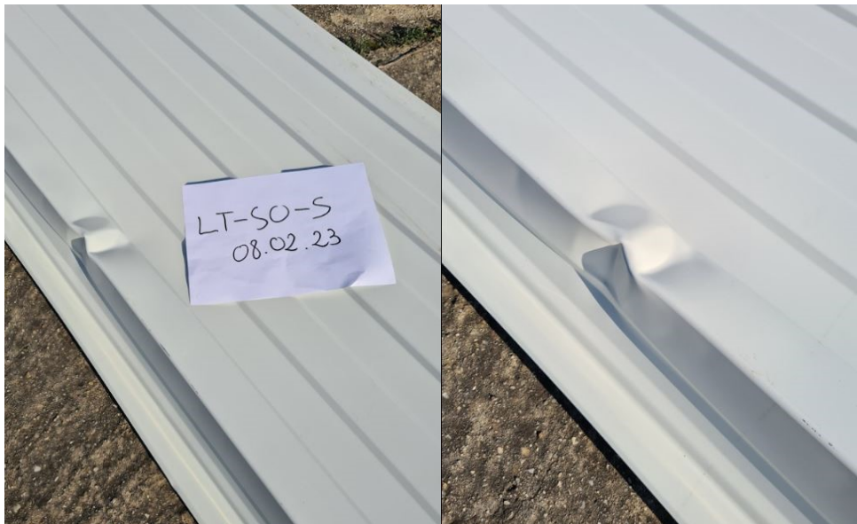
Figure 3.51 Detail of the failure zone: local buckling of the area under compression
