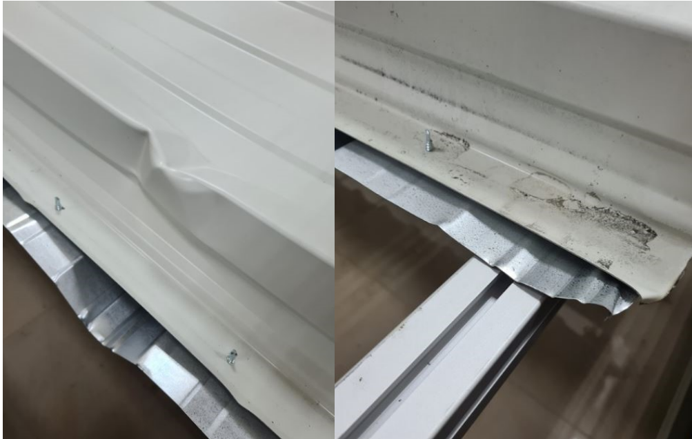
Figure 3.55 Detail of the failure zone of the liner tray: local buckling of the wide flange interacting with local+distortional buckling of the web (left) and flattening of the corrugated steel sheet in the support area (right)
